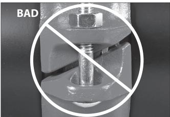
6. Visually inspect the bolt pads at each joint to verify that metal-tometal contact is achieved across the entire bolt pad section. Equal and positive or neutral offsets shall be present at each bolt pad, in accordance with step 5.
