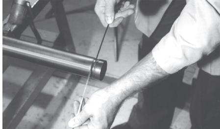
4. After dismounting the tool from the pipe, check the groove diameter to ensure that the groove meets specification.
